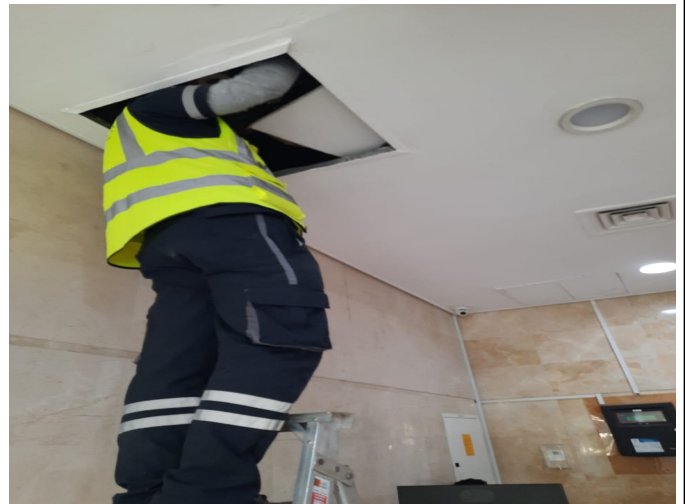
ASFM inspected reception and lift lobby above ceiling
