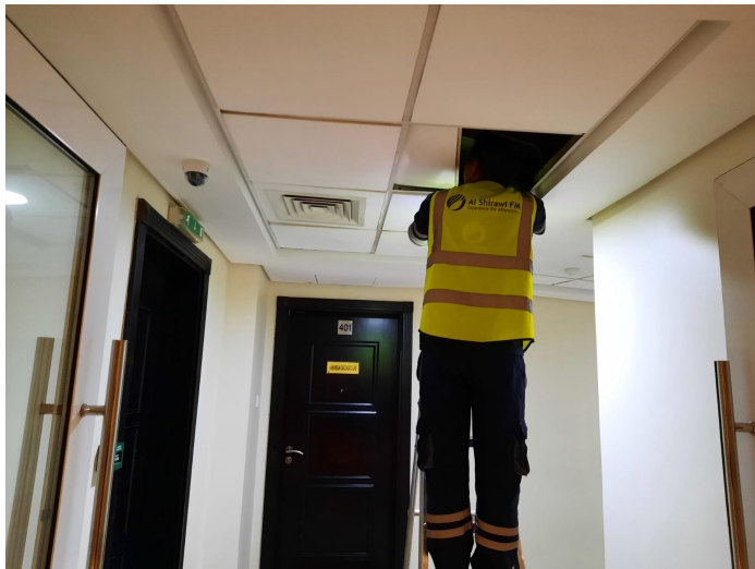
ASFM inspected 4th floor above ceiling
