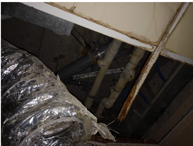
Bidet drain pipe leaking at Apt 116 master washroom ceiling
